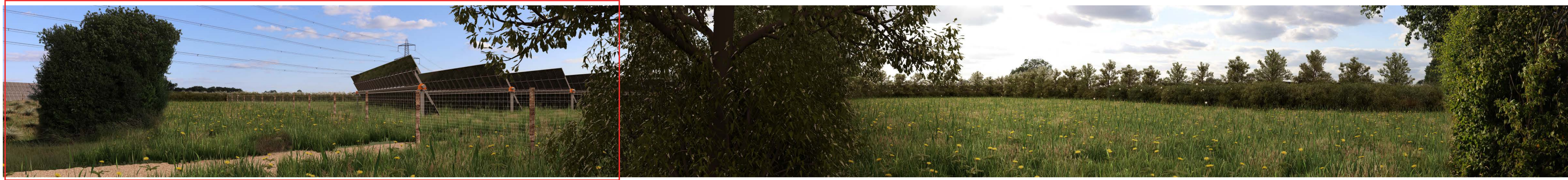
Site Context Photograph (1 of 2)
